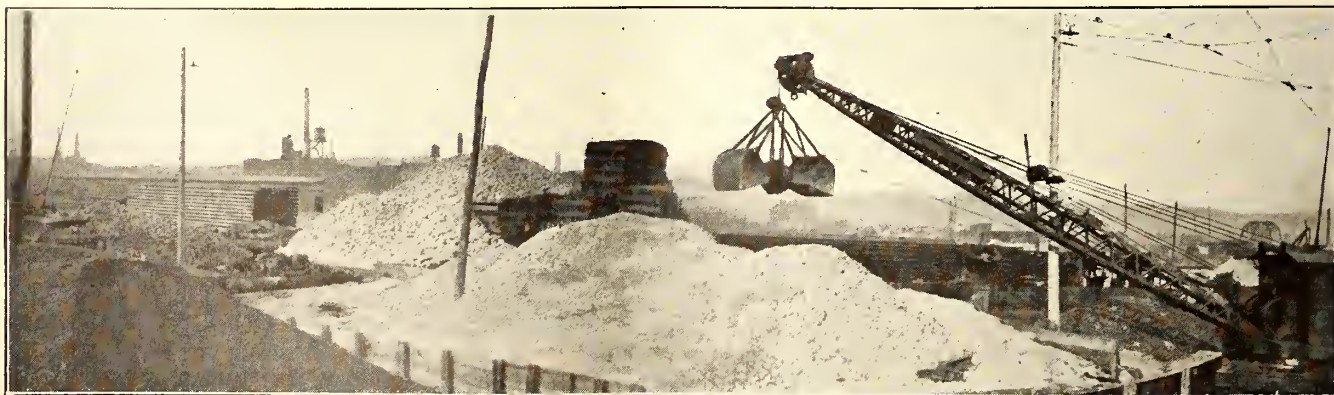
VIEW SHOWING HOW MATERIALS CAN BE STORED IN LARGE QUANTITIES BY USE OF THE LOCOMOTIVE CRANE
